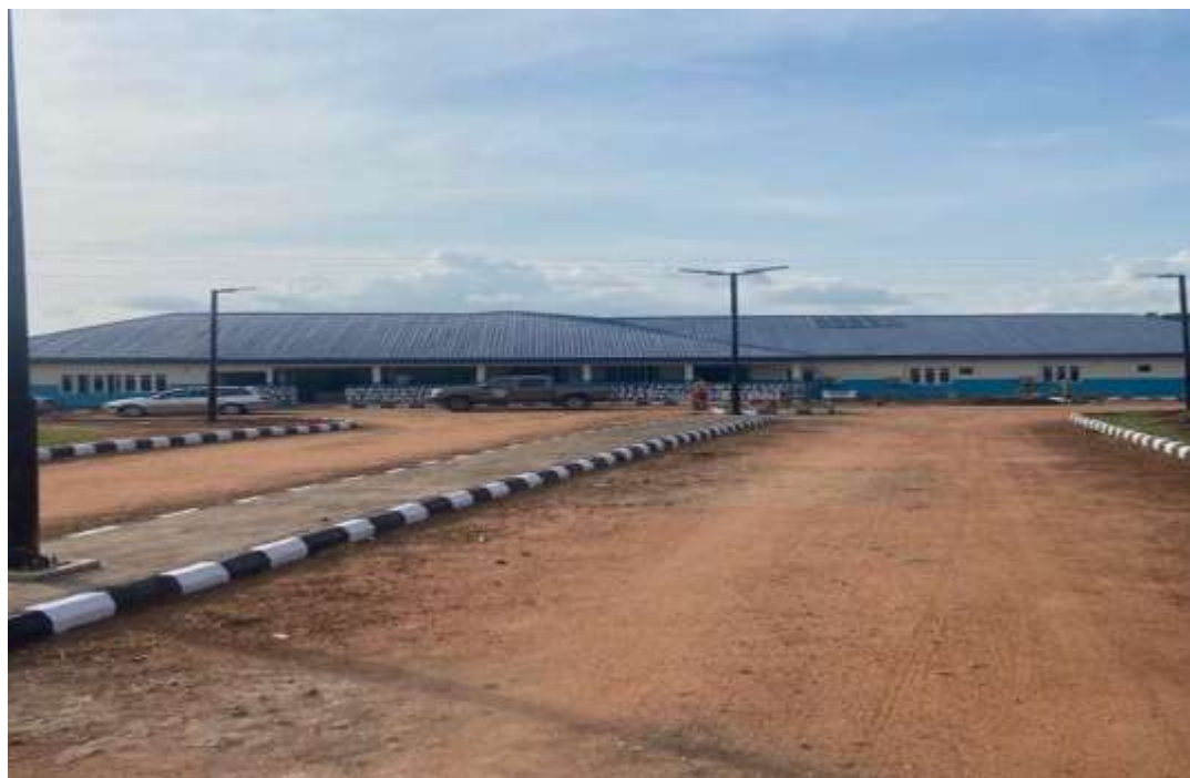
(Pictures of G.H.Tede after Renovation).
