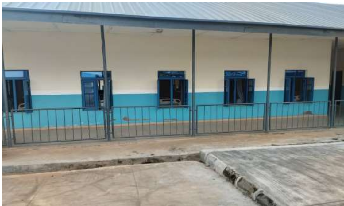
(Pictures of G.H. Aremo after Renovation)
